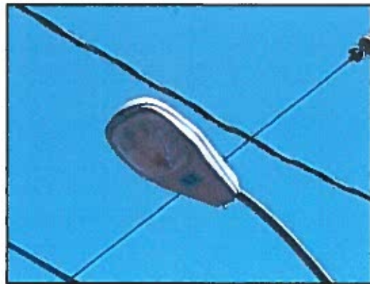
Drop dish Cobrahead 175w MV
